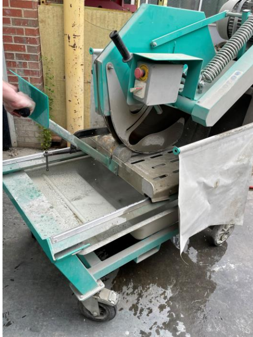
Figure B.7: Deck concrete removal by saw-cutting.
