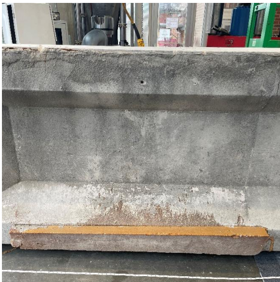
Front end spall repair (right side)
