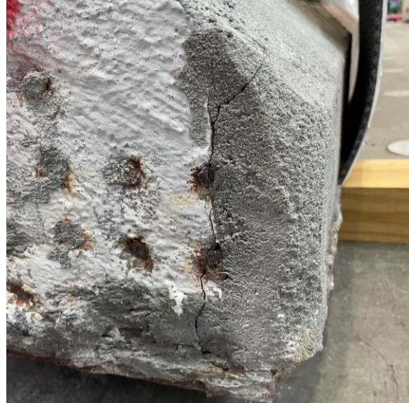
Front corner spall repair (right side)
