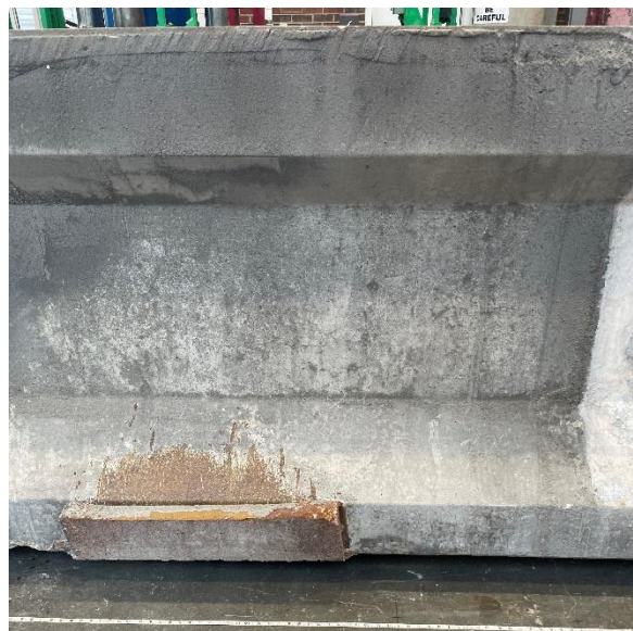
Front end spall repair (right side)
