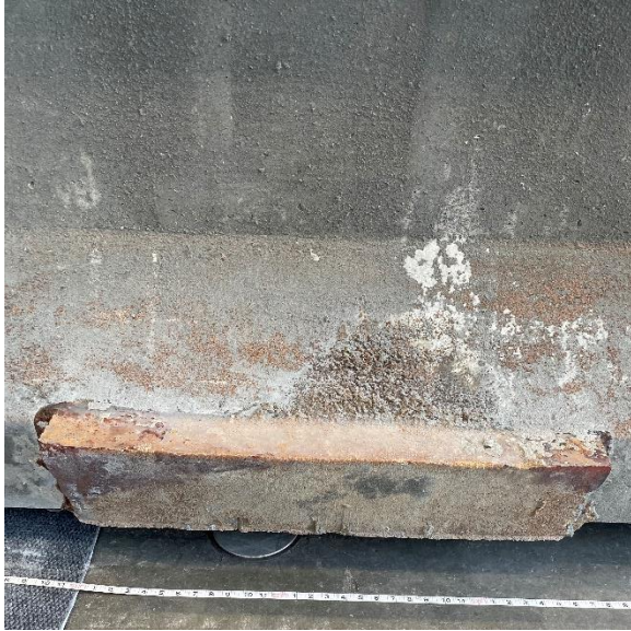
Spall repair (left side)
