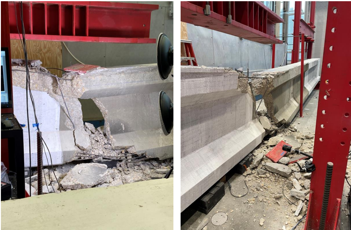
Figure C.2: Photo of BTE1 after failure.
