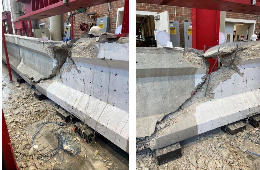
Figure C.22: Photo of BTE2 after failure.
