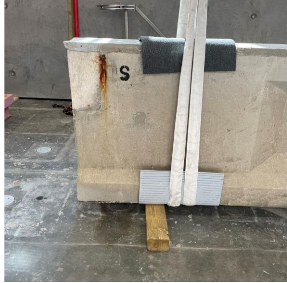
Rear end grouted hole (left side)
