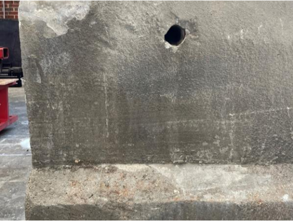
Rear end core hole (left side)
